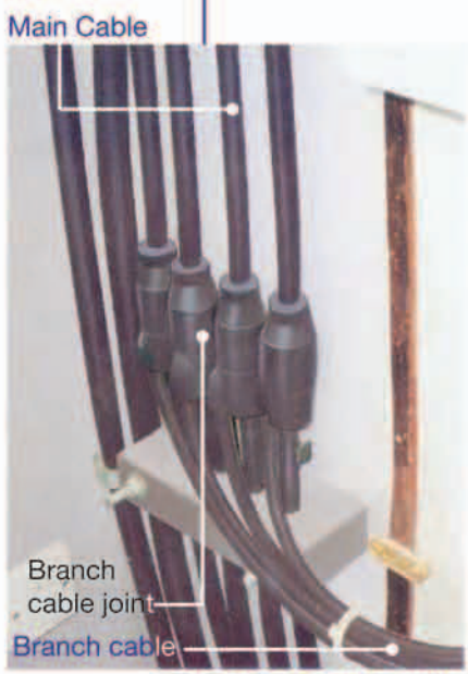
Branch cable joints with fixing and clamping apparatus
